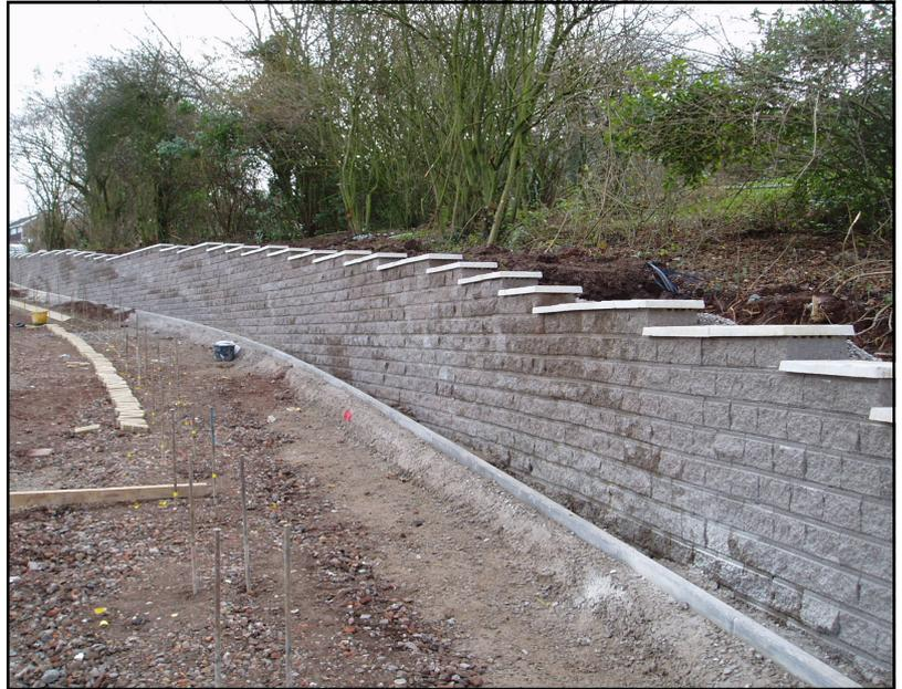
The upgrading and widening of this suburban highway sees Leromur in use to create new retaining walls alongside the footpaths. It can be difficult to gain an impression of gradients from a single photograph but hopefully this one tells its own story.
